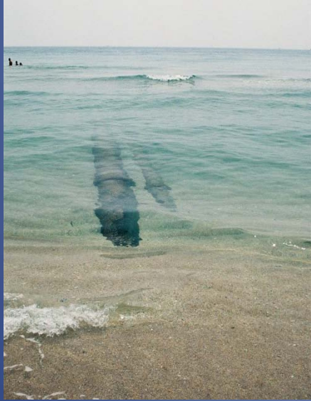
Illegal A/C drainage pipes
